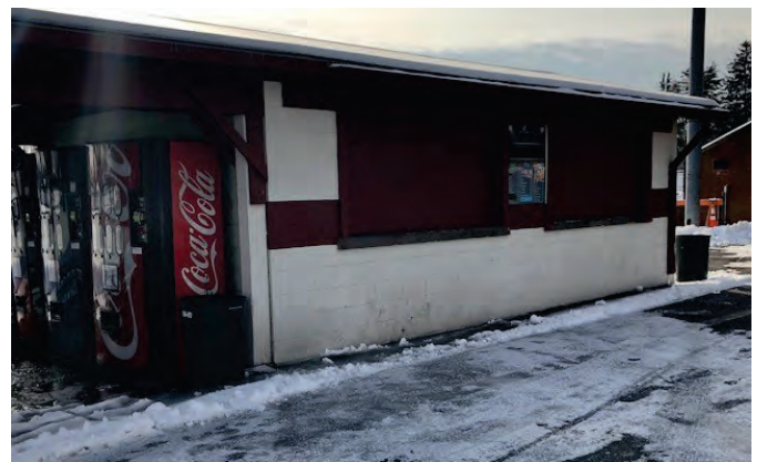
Existing food vending facility
