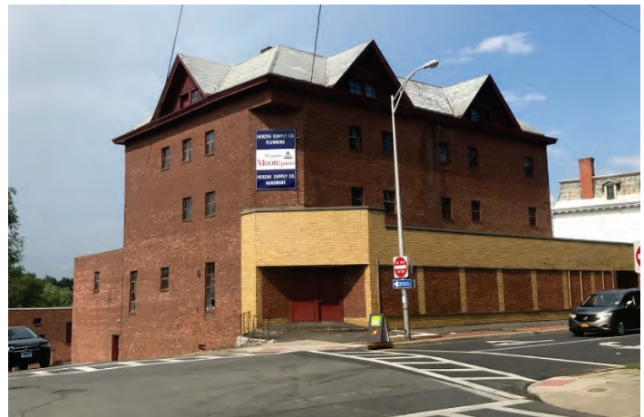
Mostly-vacant warehouse, formerly occupied by the Herzog Supply Co.
