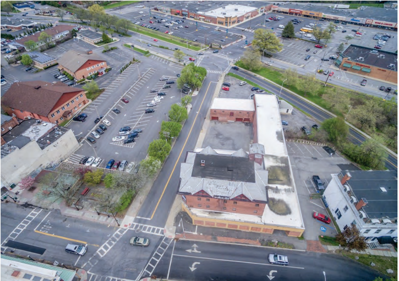
Aerial view of the Project Site
