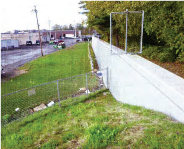
Protected side of the levee and flood wall, looking west
