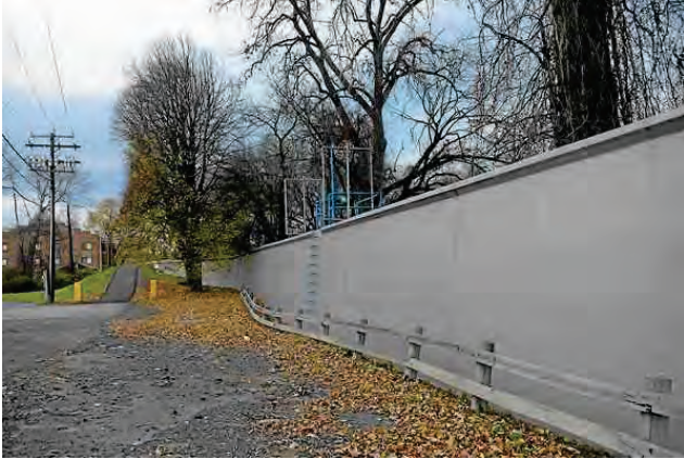
A look at the flood control wall as seen behind Mac Fitness at the Kingston Plaza
