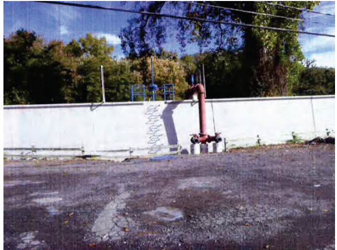
Protected side of the flood wall
