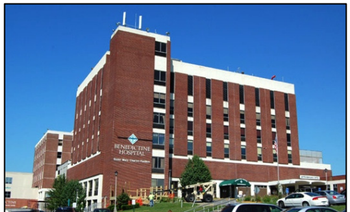
Above (top to bottom): View of City Hall that is adjacent to the Kingston Hospital; view of the Ulster Performing Arts Center on Broadway and view of Benedictine Hospital on Mary's Avenue. The existing industry/activity clusters within Midtown should be encouraged to grow further.
