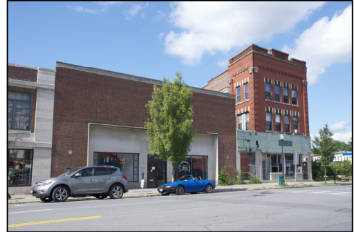
Above: View of the underutilized buildings along Broadway in Midtown.
