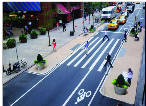
Above: Example of complete street and road diet concepts. NYCDOT (from www.spur.org )
