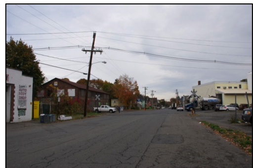
Above (top to bottom): View Broadway looking northwest from the railroad overpass; view of active CSX railroad bridge that crosses over Broadway (West Shore Railroad Line); and view looking north along O'Neil Street in the vicinity of Boice's Dairy and the defunct Delaware & Ulster Railroad yard. A visitor to Midtown experiences a corridor, neighborhoods and former manufacturing nodes that appear, in certain places, past its prime and weary to the eye.
